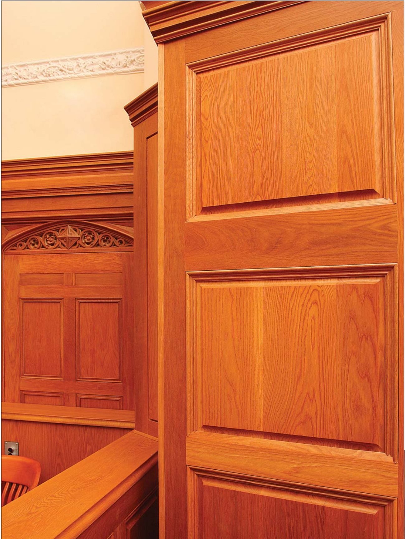
THIS CORNER OF THE COURTROOM illustrates the merging of the old existing White Oak panels and the new panels.
